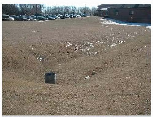
Infiltration basins are designed to collect stormwater from impervious areas and provide pollutant removal benefits through detention and filtration
